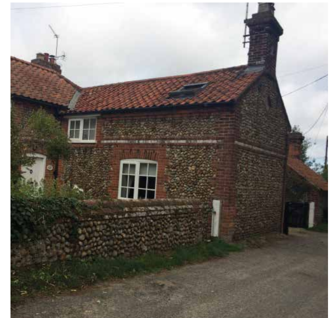
Brick and flint cottage and garden wall against roadside. White flint course detail used on No.3 The Street
