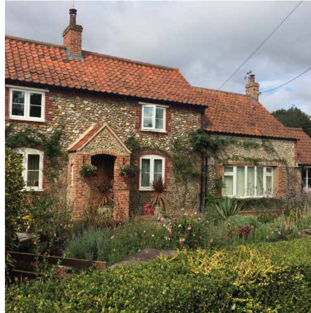
The Old Forge Cottage typical of the area with the use of red brick, flint and terracotta pantile roof.
