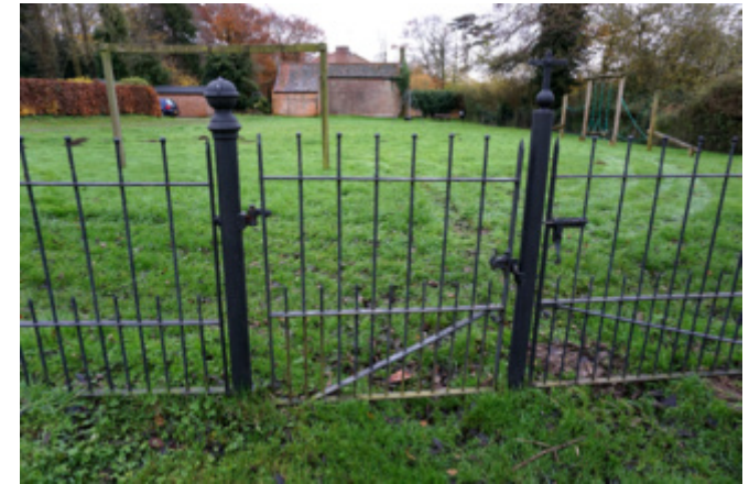
Metal gate and railings to the graveyard
