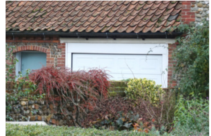
Modern garage doors inserted into historic fabric
